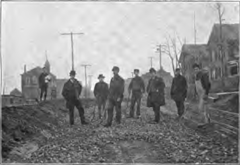
Sayreville road, Middlesex Co., laying first course.
